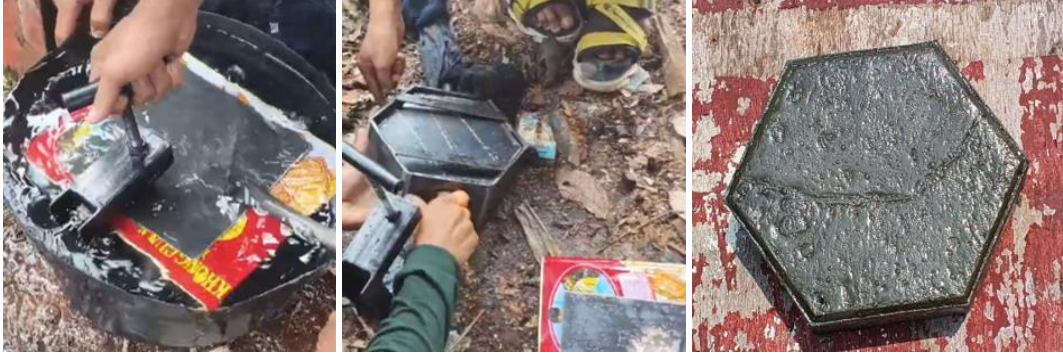
Gambar 2. Proses Mencetak Paving Block
